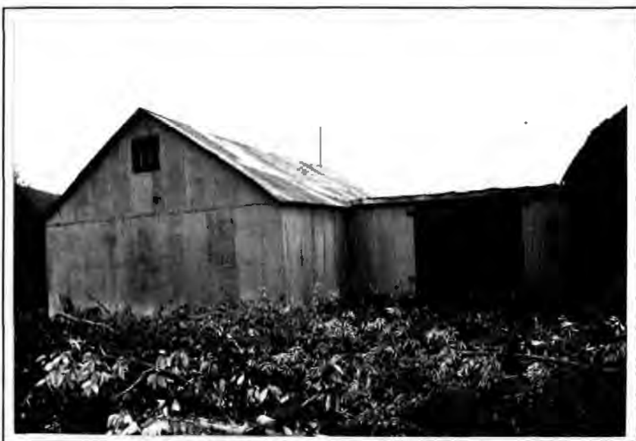
Figure 41. The Donnelley Pipe Warehouse, 1993. The view is looking northeast.
